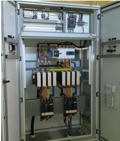
MDB Busbars State of the arts ATS-MDB Automated Panelboard MDB Busbar
