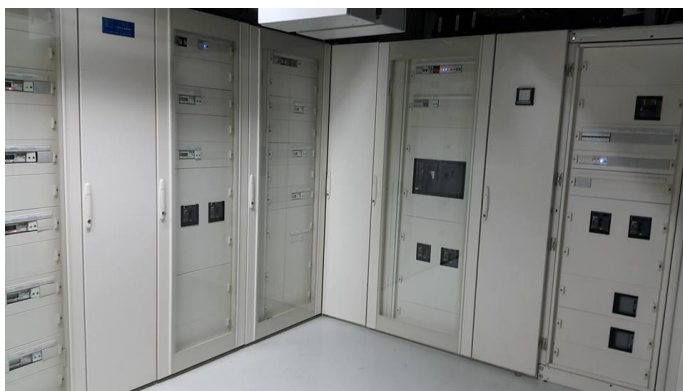
ATS and MDB Panel Prisma-P Form-3 with Power Metering
