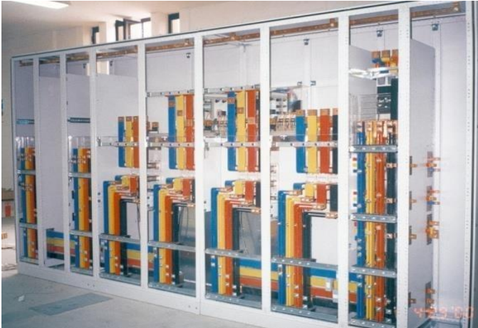
MDB Busbars State of the arts ATS-MDB Automated Panelboard MDB Busbar
