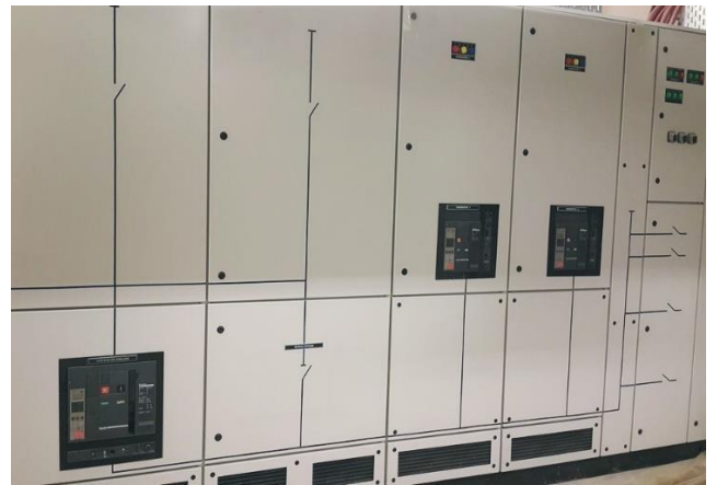
Totalizing Panel 2500Amp Form-3
