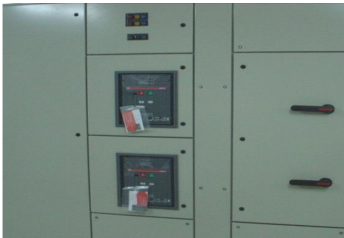
Totalizing Panel 2500Amp Form-3B
